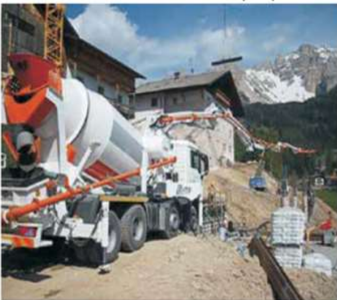
Truck Mixer with Concrete pump
